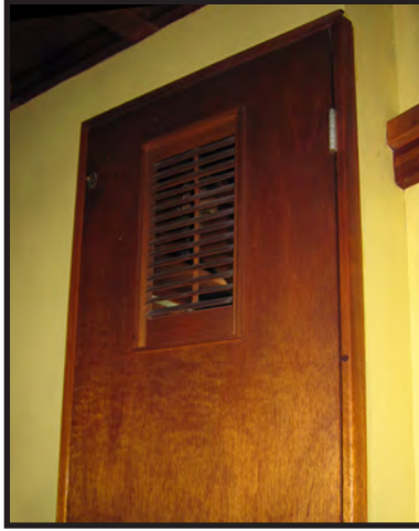
The door to Larry's cabin (and the bow cabin).
